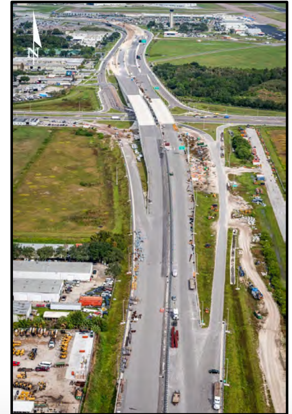
New SR 686A toll road at Ulmerton Road interchange
