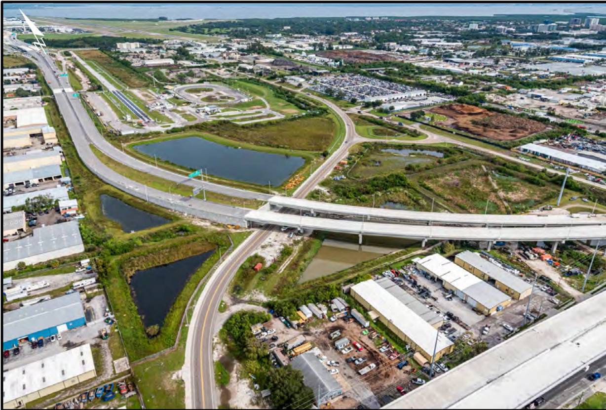
New SR 686A toll road between 118 th Avenue. N and Ulmerton Road
