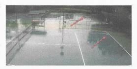
Some staining from the dirt and tree & shrub materials along with some debris adherence remained. The adherence of even small particles may disturb play. The surfaces are effectively more vulnerable due to the combination of the water-born debris with the continuing extraordinary heat.
